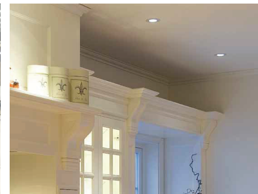
ILL. SOLAR LIGHT SPOTS
