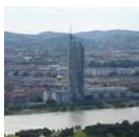
Millenium Tower Wien-Østrig
